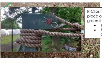
R-Clips holding bar in place on both sides of green frame.
